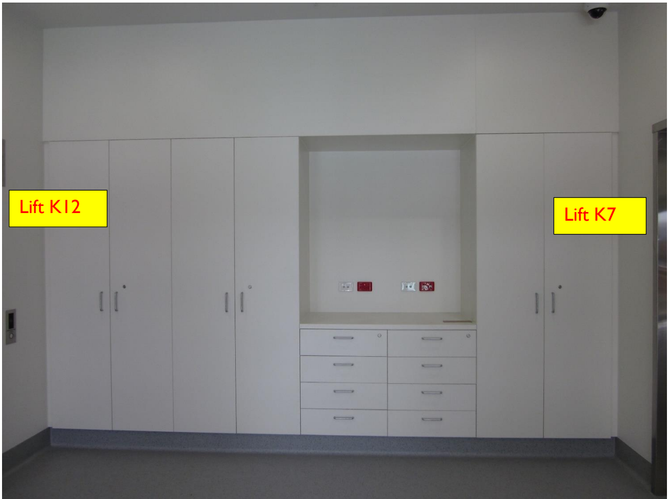
Figure 12 – Heliport Lift Lobby Equipment – Western Wall – Equipment Storage Cupboards
