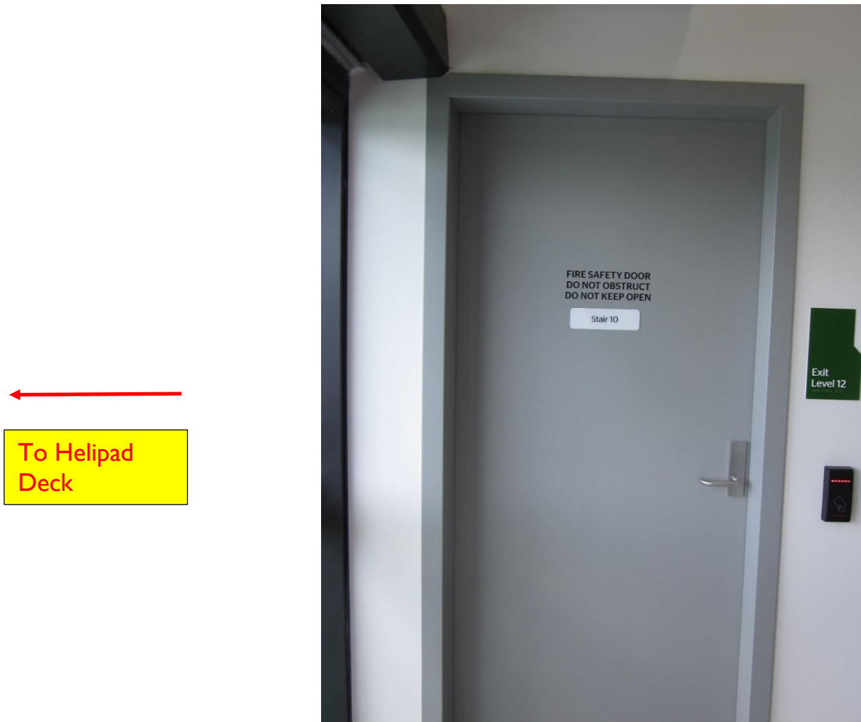
Figure 21 – Stairwell 10 Entry (inside Heliport Lift Lobby)
