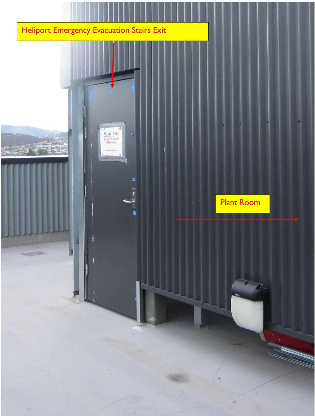
Figure 25 – Heliport Emergency Evacuation Stairs – Exit at Plant Room Level
