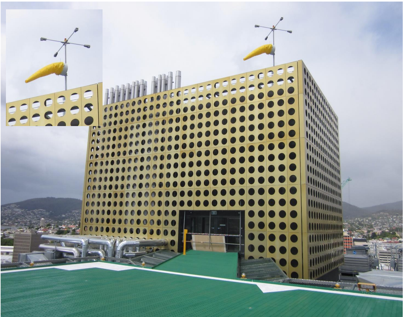
Figure 1 – Location of Primary Illuminated Wind Direction Indicator Relative to Heliport
