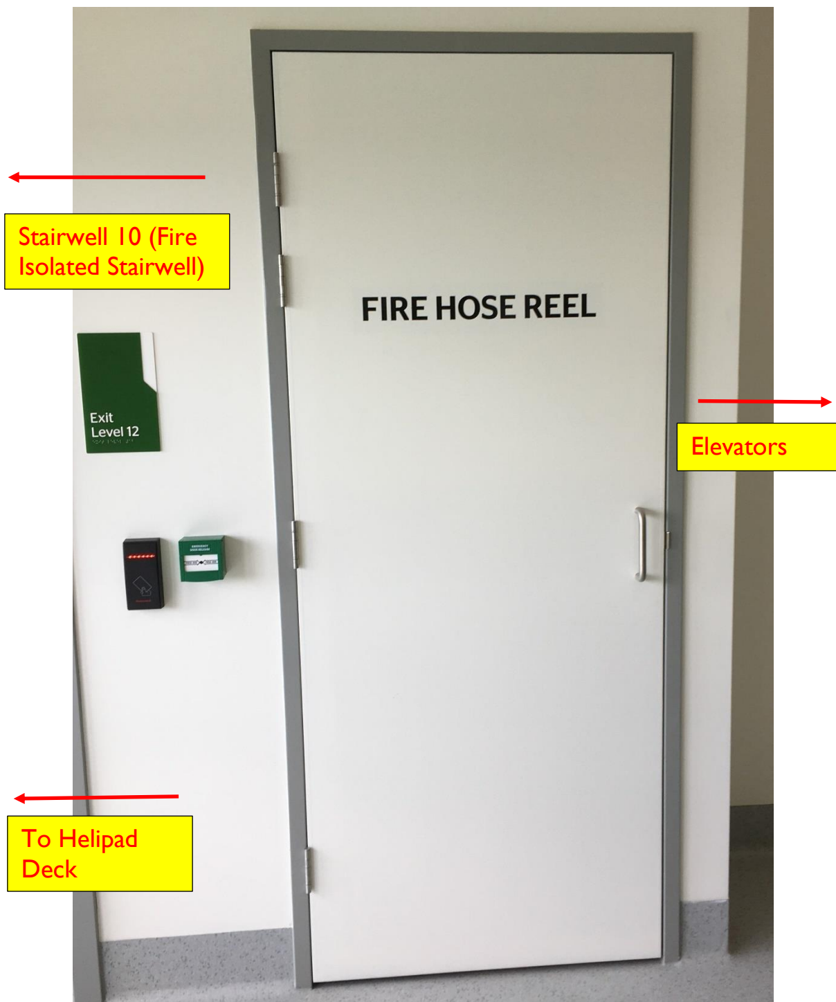
Figure 11 – Heliport Lift Lobby Equipment – Southern Wall – Fire Hose Reel
