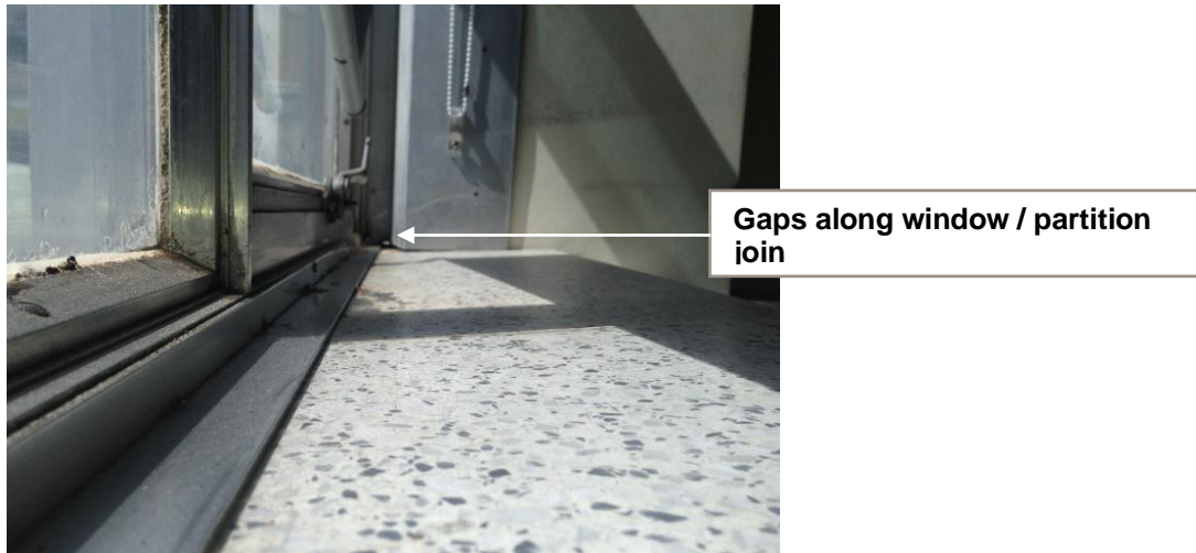
Figure 9 –Window / Partition Join, Building H
